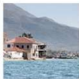
Highest corrosive environment
